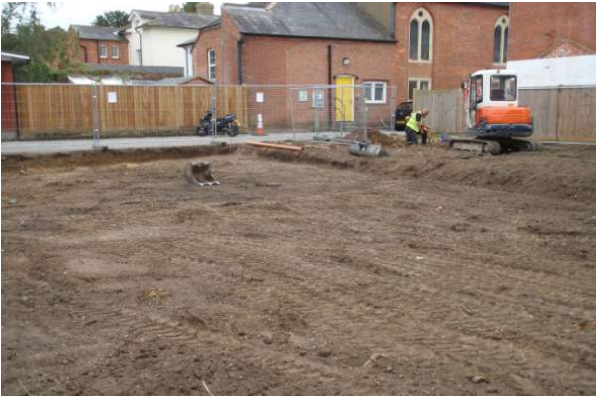
Plate 2. Phase 1, view of the site after topsoil strip (looking south-west)
