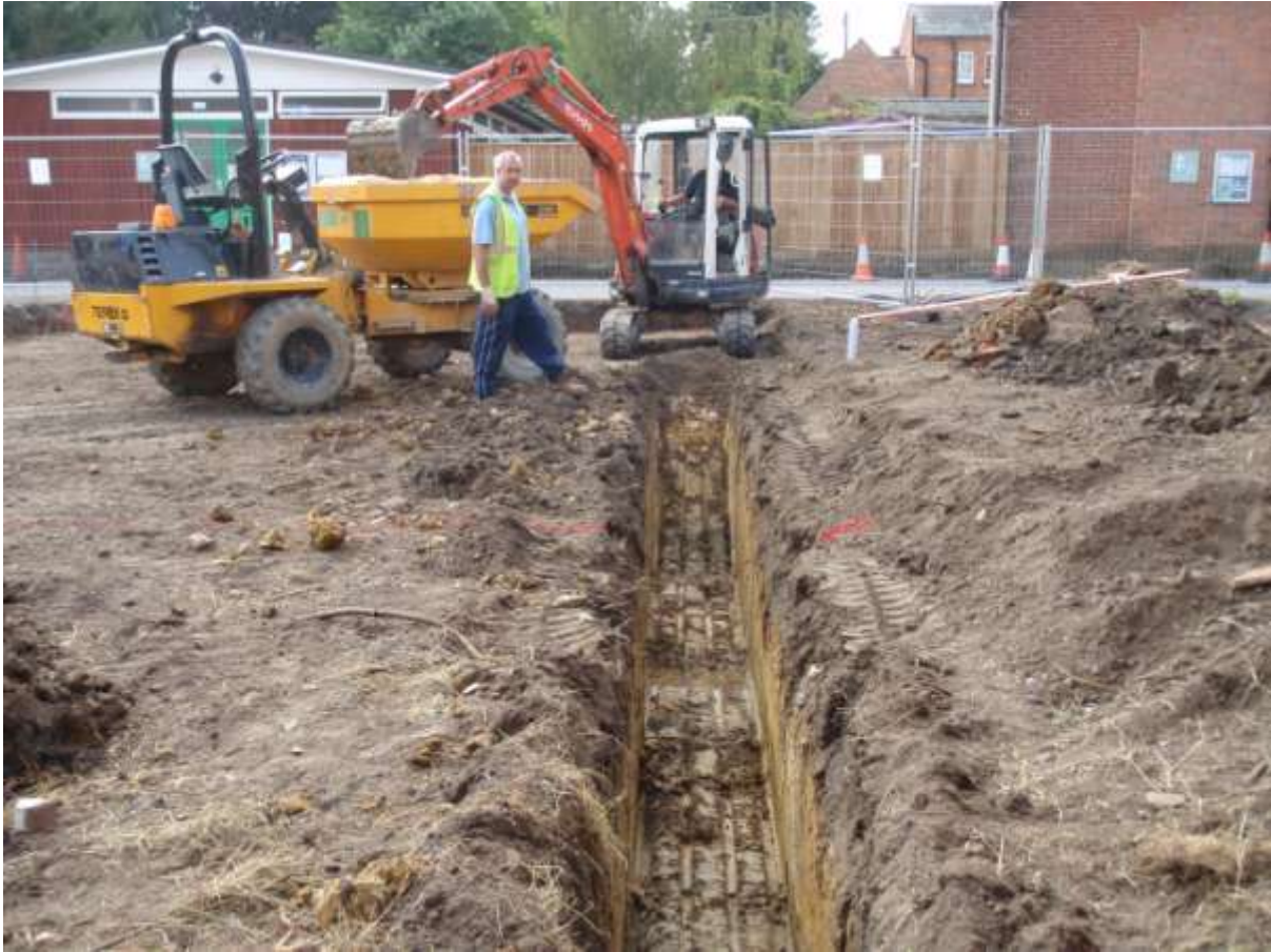
Plate 4. Phase 2. Trenches being excavated (looking SSW)
