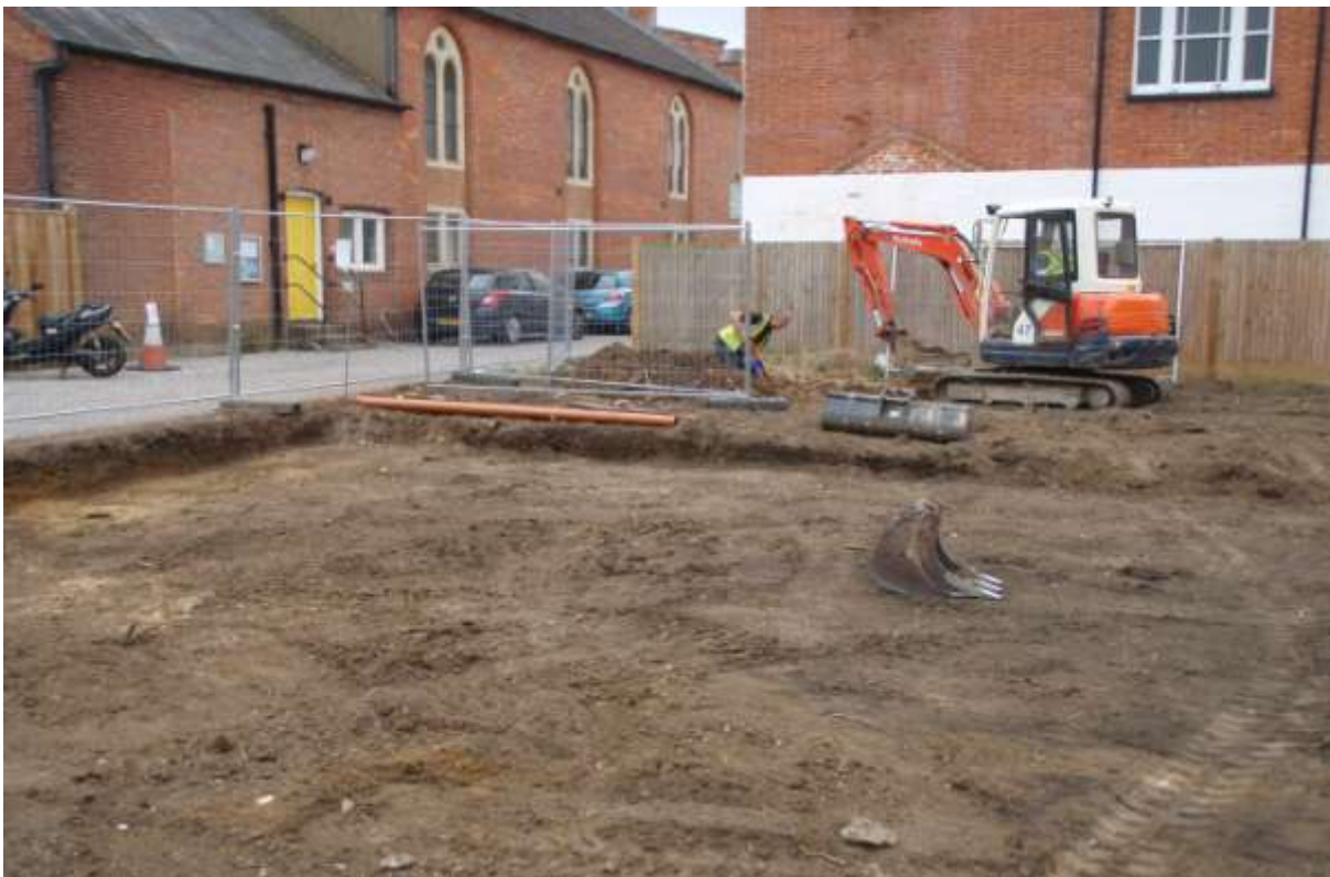
Plate 3. Phase 1, view of the site after topsoil strip (looking west)
