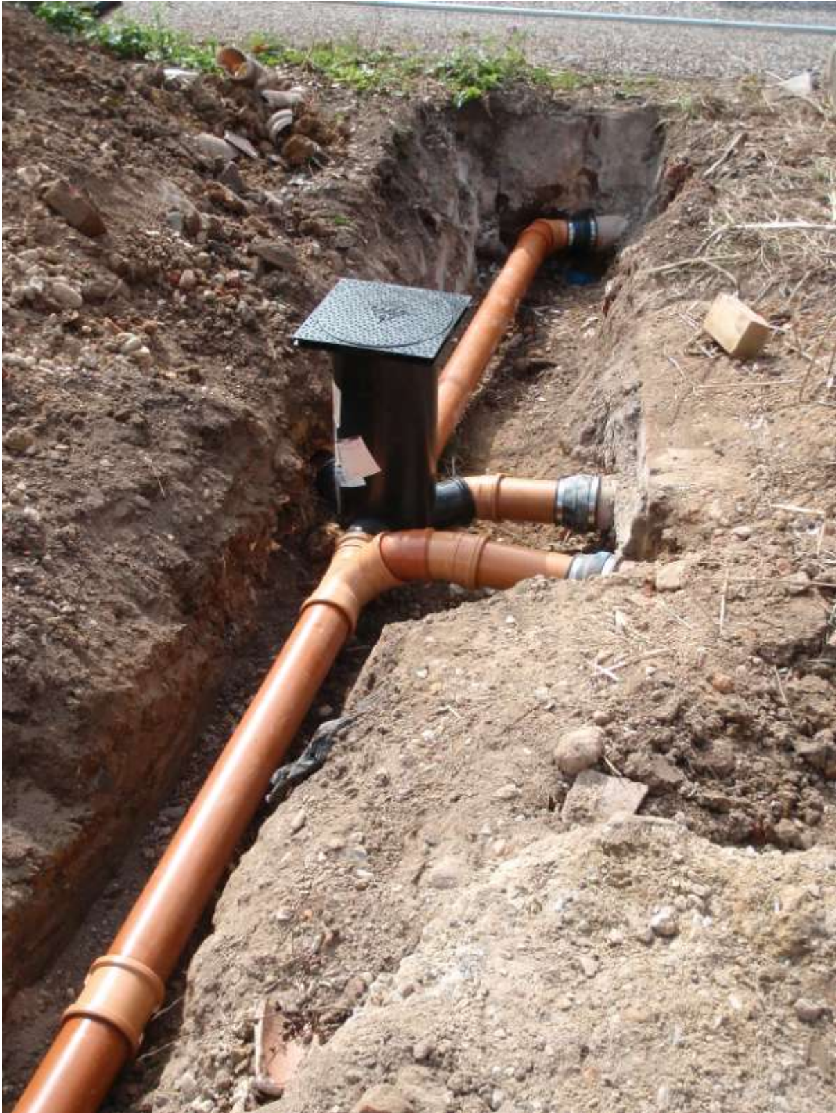
Plate 6. View of site showing service trench (looking SW)
